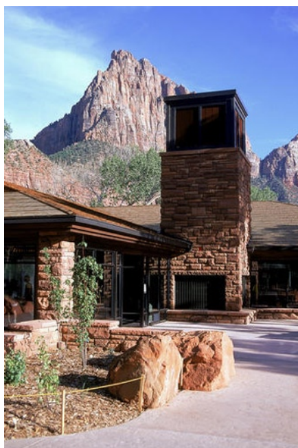
Cool tower at Zion Visitor Center
