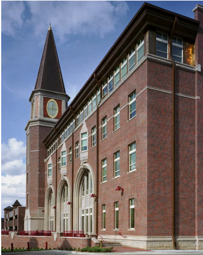
University of Denver's LEED-NC Gold College of Law Building Featured in the November/December 2005 issue of CBG
