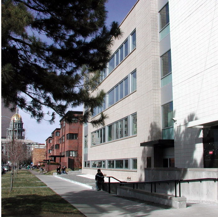
State of Colorado Dept. of Labor and Employment Addition Architect: David Owen Tryba Architects
